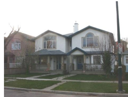
Example of a duplex with a recessed party wall, creating the illusion that they are two separate dwellings.
