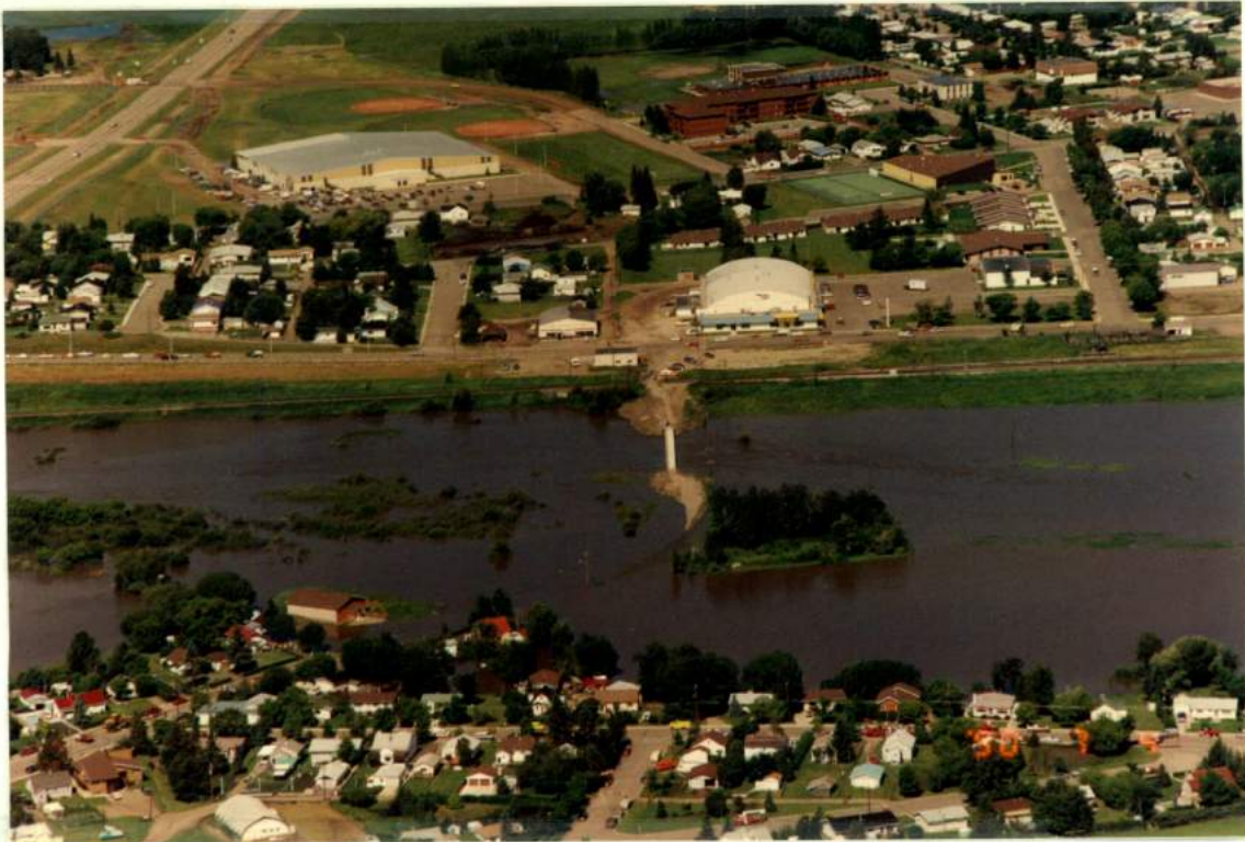
PLATE A-5 PEDWAY AT SECTION X13, LOOKING WEST
