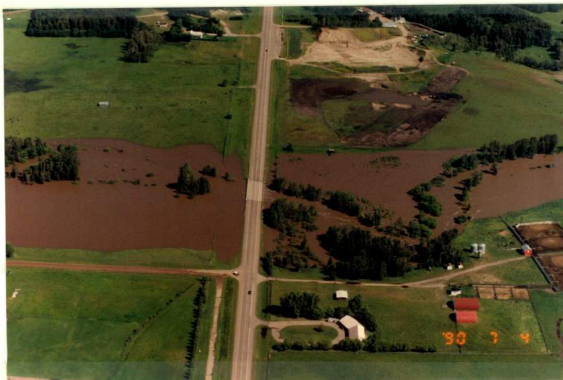
PLATE A-8 HIGHWAY 2A BRIDGE AT SECTION X 21, LOOKING NORTH
