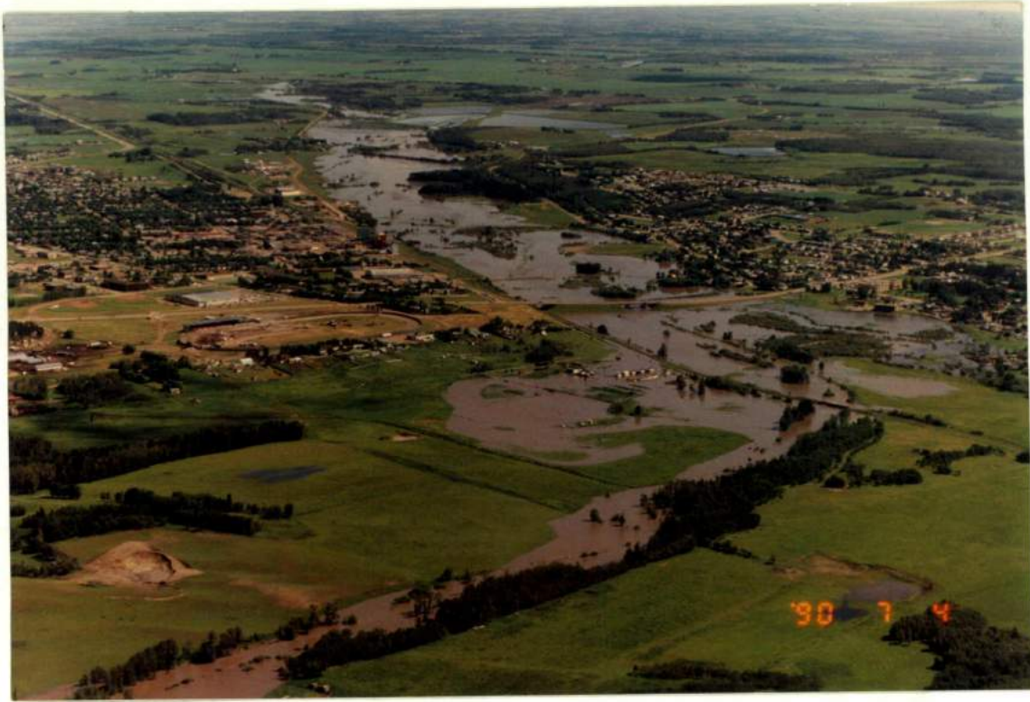
PLATE A-1 FLOOD OVERVIEW LOOKING DOWNSTREAM FROM SECTION X19
